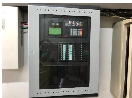
Fire Alarm Control Panel: FCP
